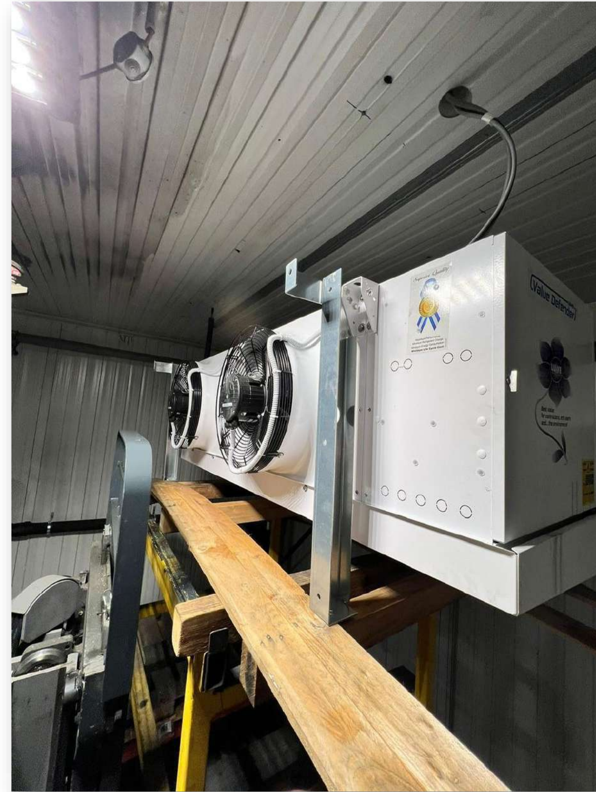
Lifting MT evaporator
